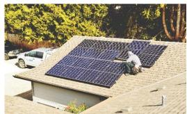
The proposed system offers (30) 330W modules for a total DC capacity of 9.9 kW and can be expected to produce ~10,679 kWh of electricity annually. Based on your historical consumption of ~15,300kWh/year this system can be expected to cover ~40-50% of your annual energy usage.
